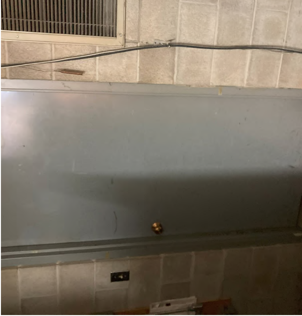
Room 100 Access Door - 3' Opening
