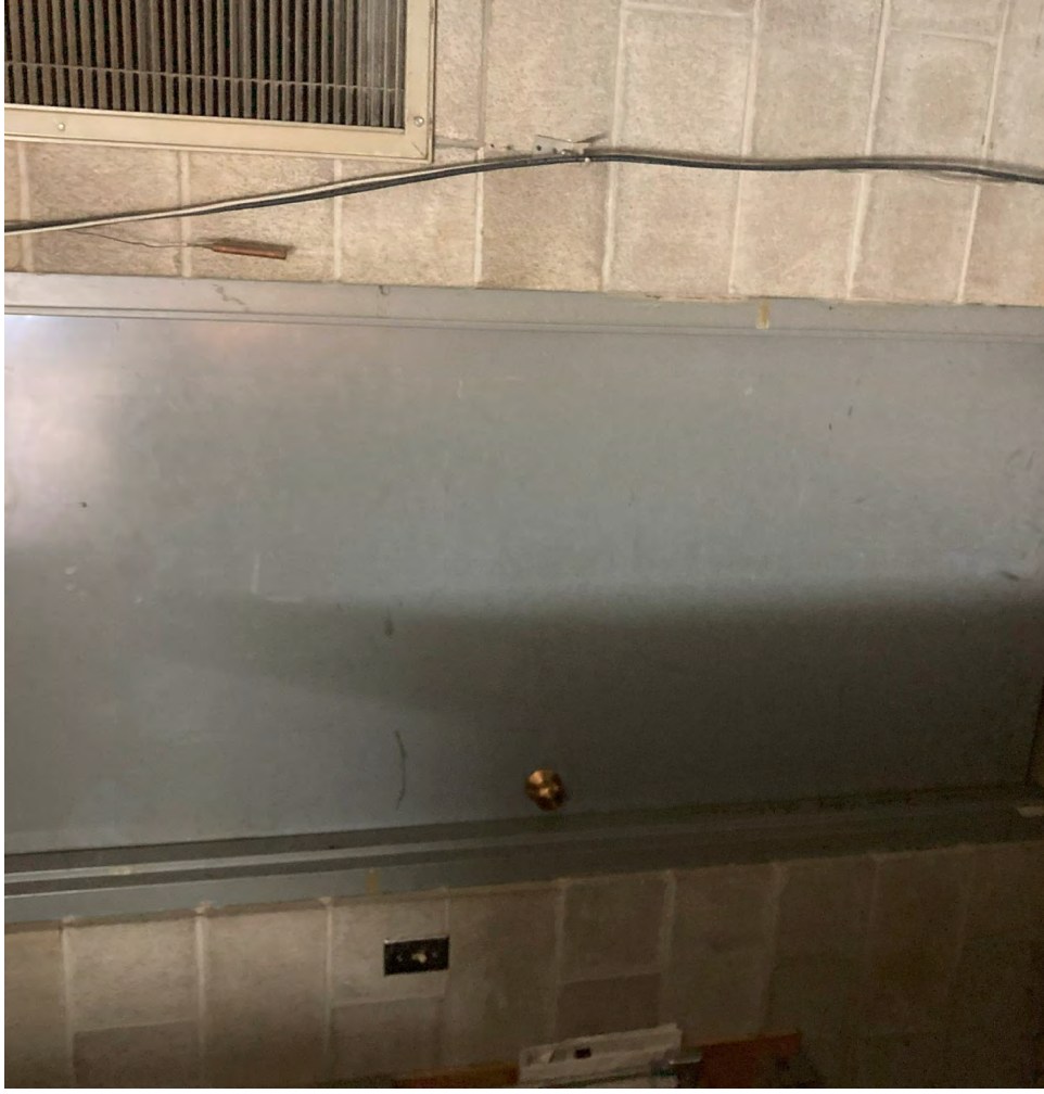
Room 100 Access Door - 3' Opening
