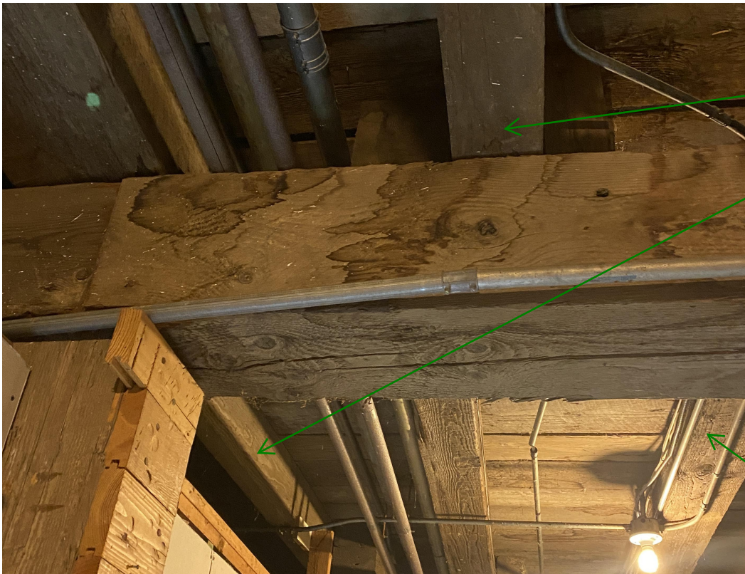
EXPOSED JOIST FRAMING IN MECHANICAL ROOM
