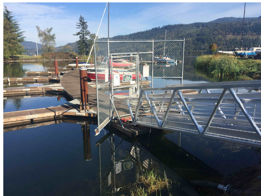
B West Dock Gangway and Gate
