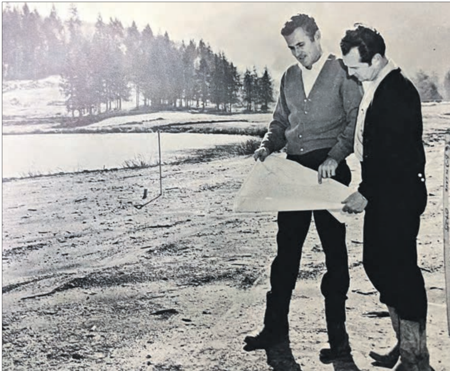
1969: Ted Robinson, left, surveying plans for the Sudden Valley course with engineer partner Don Hogan on what would become the 6th hole.
